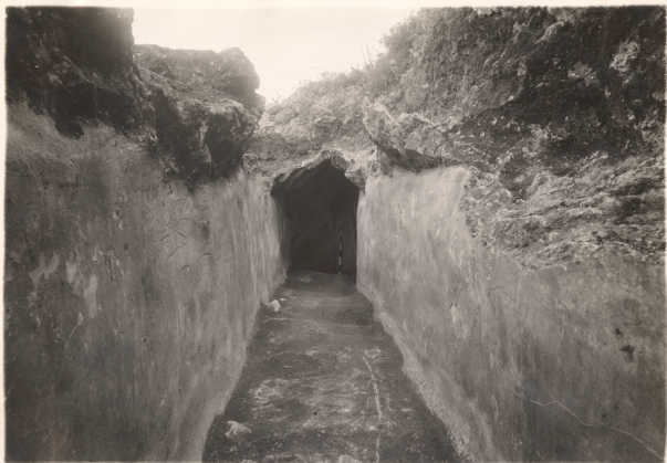
Fig. 3 Channel of aqueduct in 17-Q
