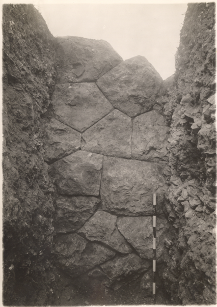
Fig. 7 Trench against back of polygonal wall in 17-Q
