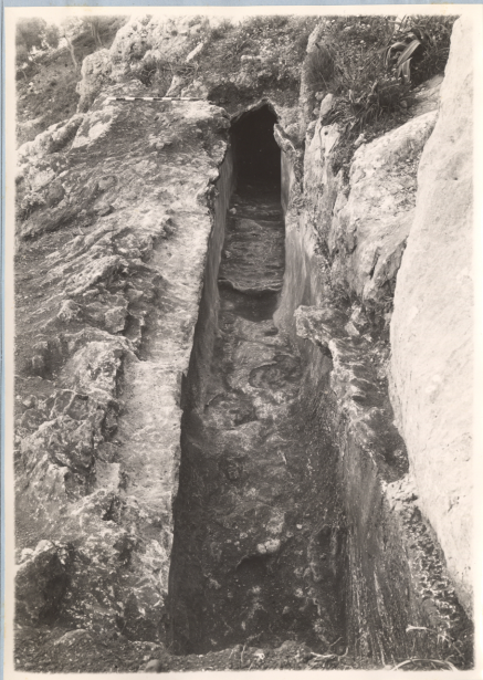
Fig. 1 General view of aqueduct in 17-Q.
