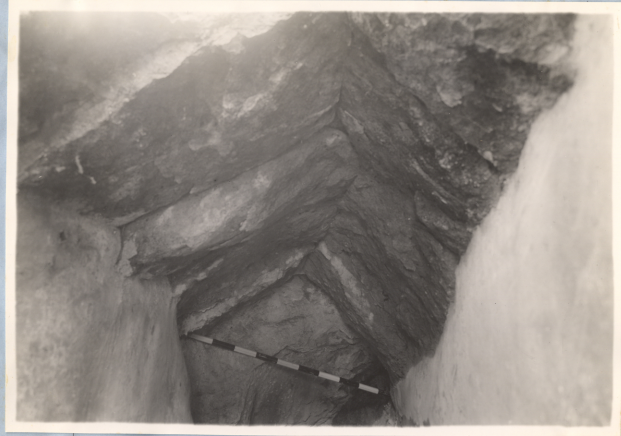
Fig. 2 Cover of channel of aqueduct in 17-0
