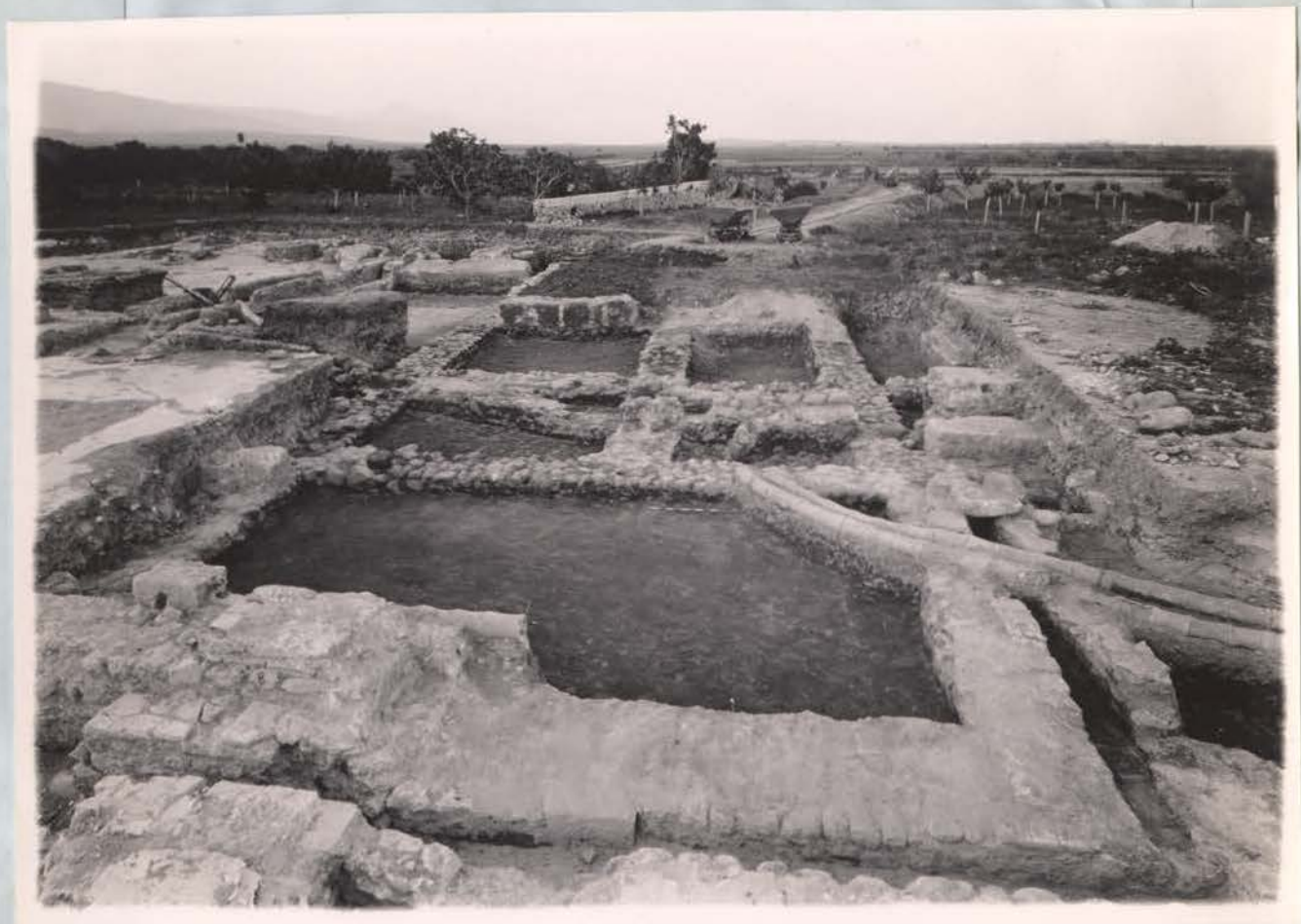
Foundation Walls, Aqueduct, and Drains East of Bath E.
