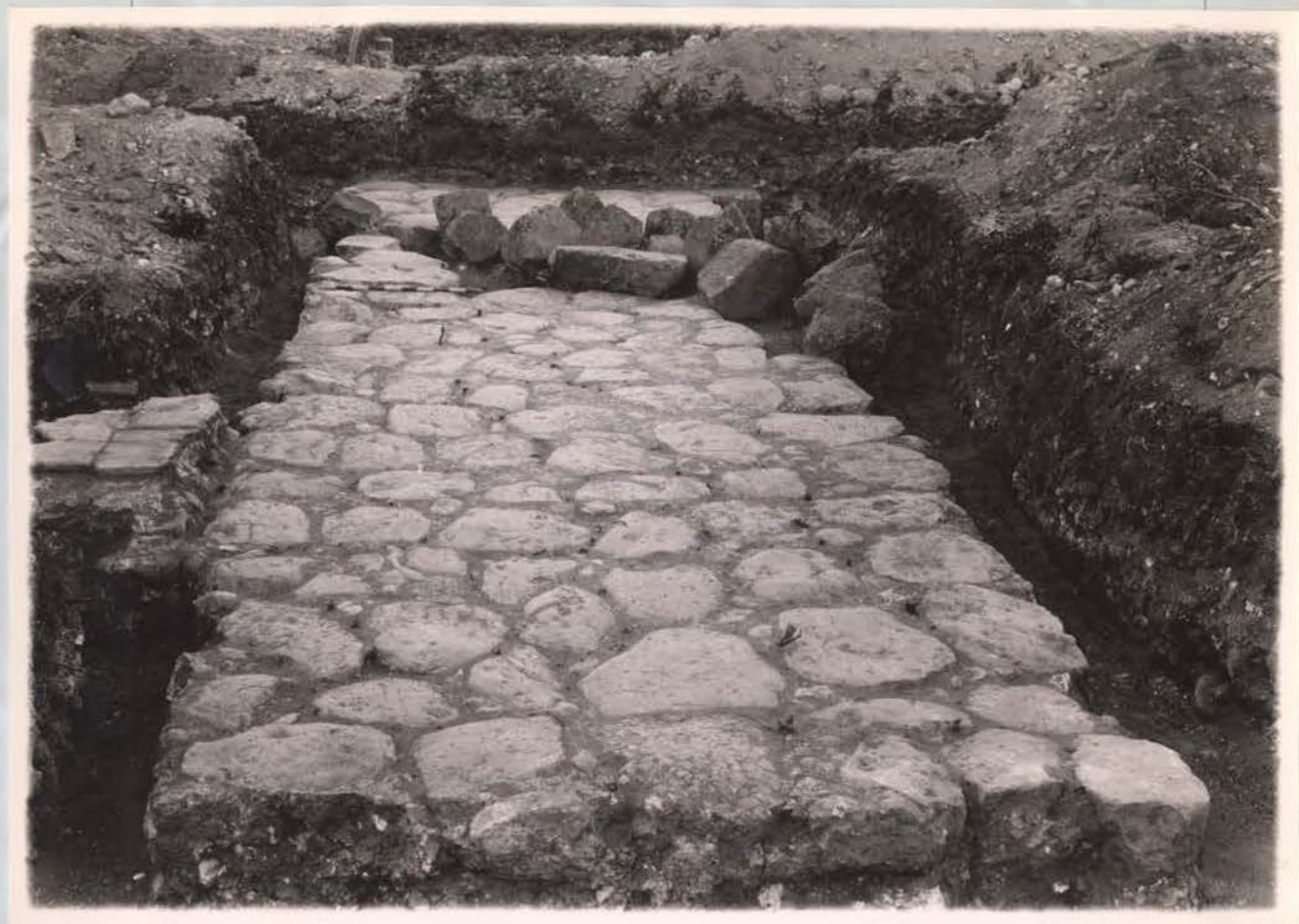
Road of Basalt Boulders near Bath E partly Destroyed by Earthquake.
